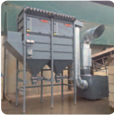
Extraction unit DUSTMAC S-66 and medium-pressure fan
