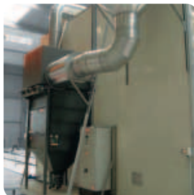
DUSTMAC filter unit on sanding station
