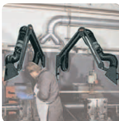
Extraction arm at a welding station
