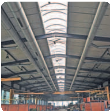
Pipeline system in the production hall
