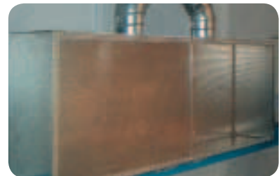
Extraction wall with perforated metal insert
