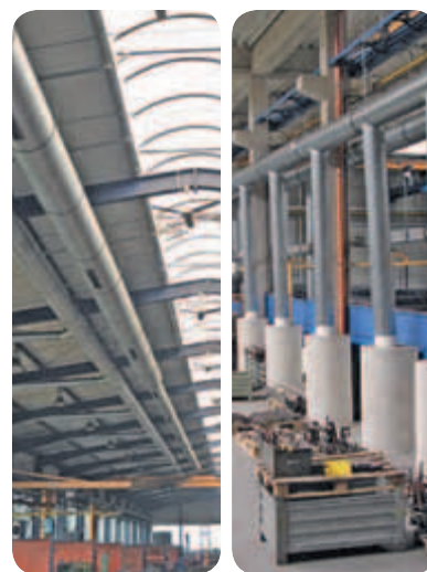
ESTA Upstream Stratification Ventilation
