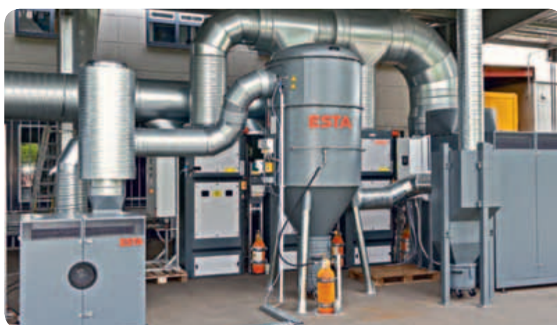
Attachment for welding fume extraction in three production halls at a car manufacturer. Several WELDEX FE cyclone filters, pre-separators and fans
