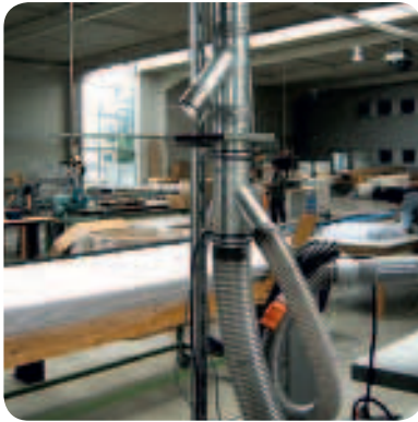
Pipe system with connection for extraction hoses
