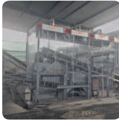
Extraction hoods over conveyor belts
