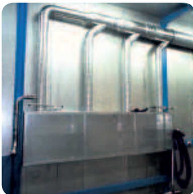
Extraction hood inside a sanding cabinet
