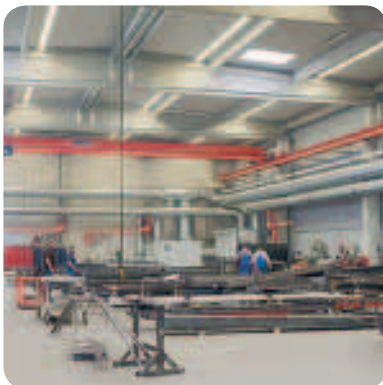
Production hall with 24 welding workplaces
