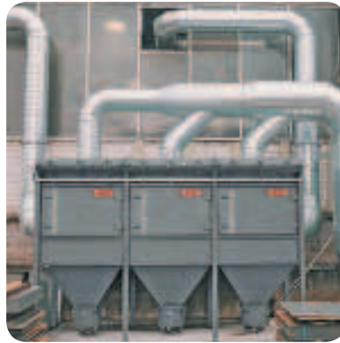
Modular filtration unit
